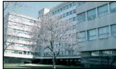
Stratton Building the TRS office from 1955 - 1966
